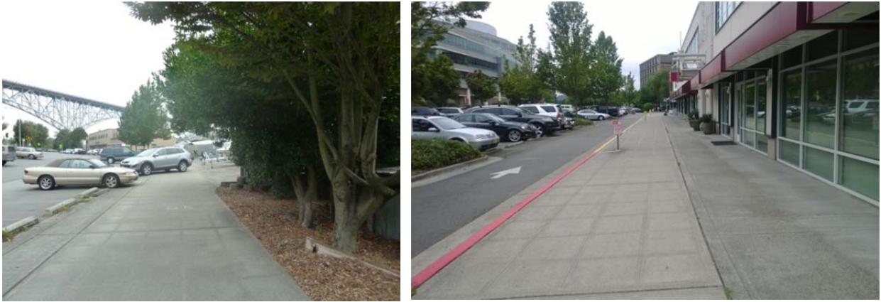
Figure 3. Conditions along east Sidewalk/Lake Union Trail.
